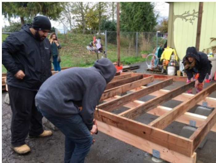
Figure 1. Attaching the foundation to the base of the tiny house.
