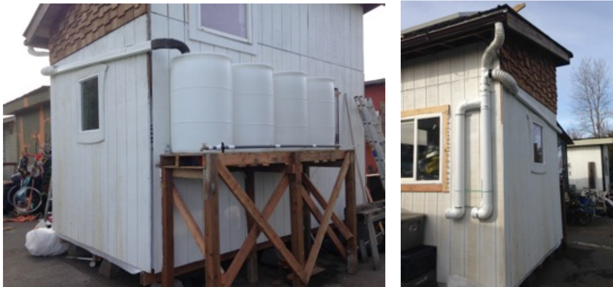
Figure 3. Gravity-fed rainwater harvesting system.
